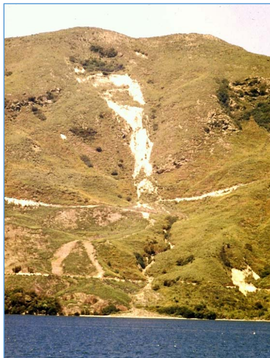
Figure 6. Erosion on Kenepuru slopes, 1962.
